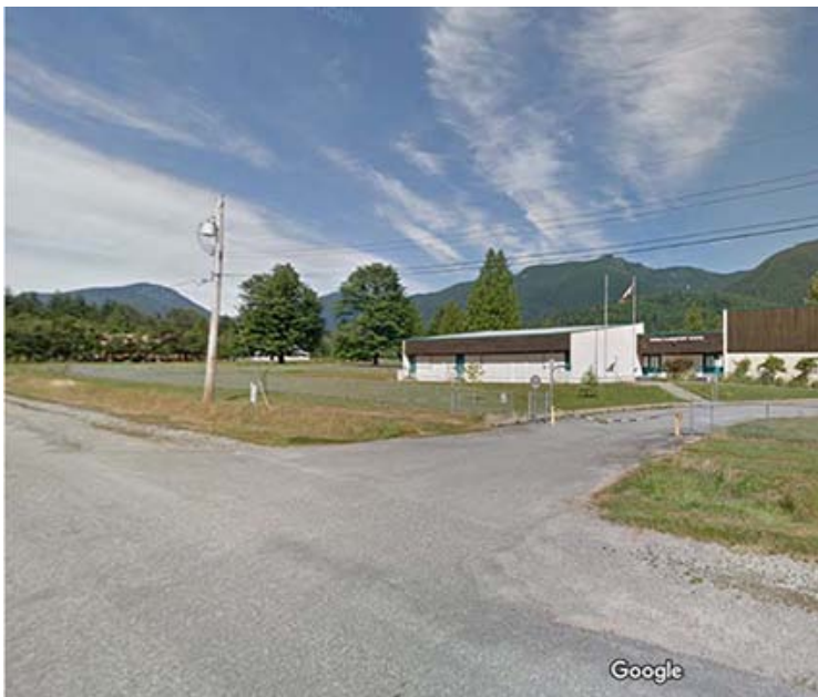
Durieu Elementary School
